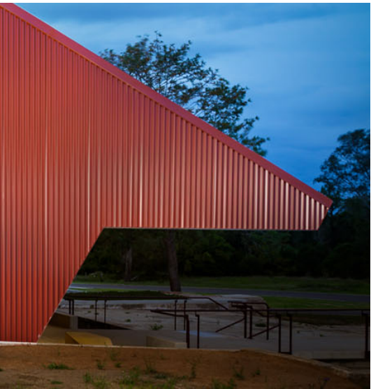
FC1/MRS - Profiled metal cladding in a heritage red type colour
